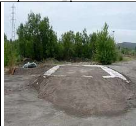
Figure 1. Experimental BOF slag road platform
